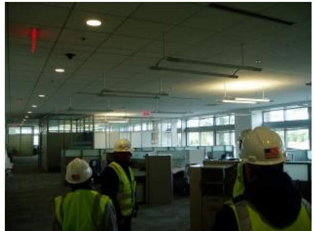
Inside Lab Office Building – Workstations – April 2009
