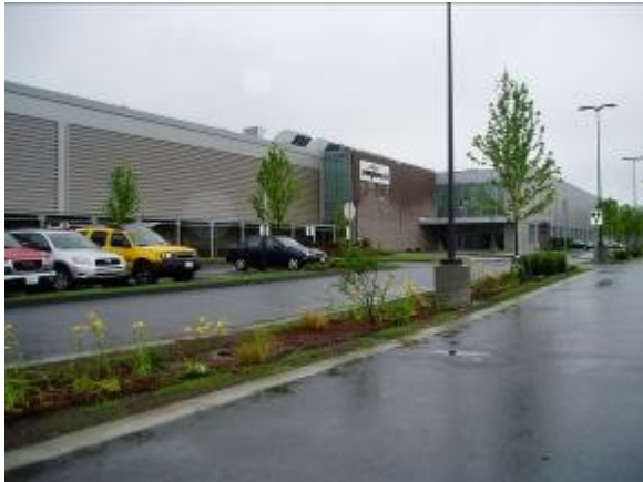
Newly landscaped front parking lot and entry
